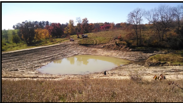
Progress on the pond at Gunderson Conservation Area.
