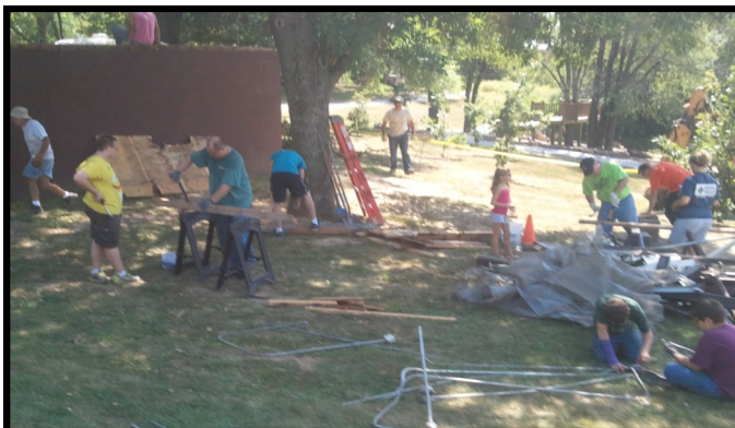
Eagle Scout project helps us tear down the old showerhouse.
