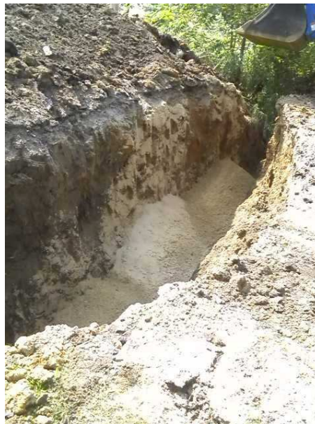
UYC Culvert Project
